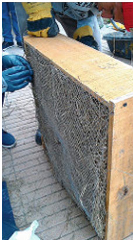
Fig. 6 Panel 2, Hay between two steel meshes
