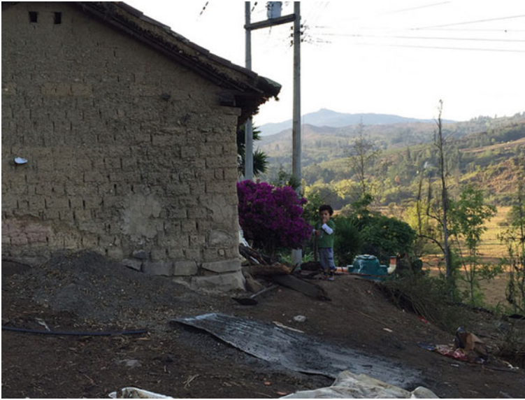
Fig. 1 The Fanny's house, old earthen bricks used in the first test
