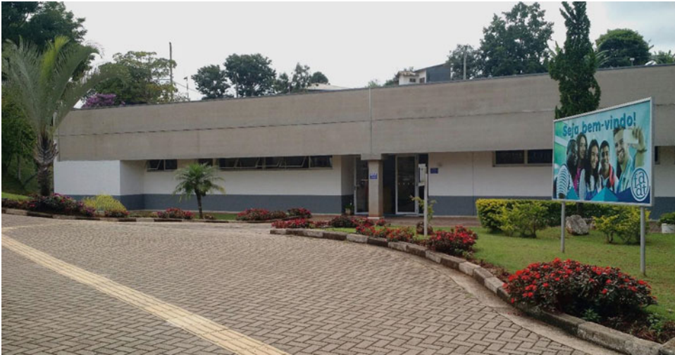
LEED O + M and Sustainable Development, Fig. 3 Administrative building of UNIFAAT. (Source: The authors 2017)
