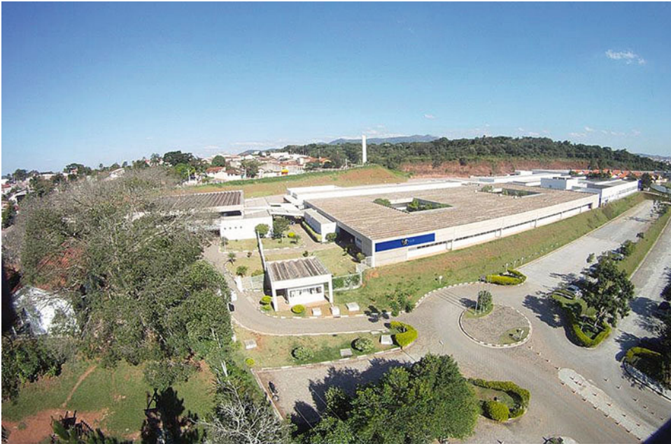
LEED O + M and Sustainable Development, Fig. 2 UNIFAAT University Center. (Source: Reproduced from UNIFAAT 2018a)
