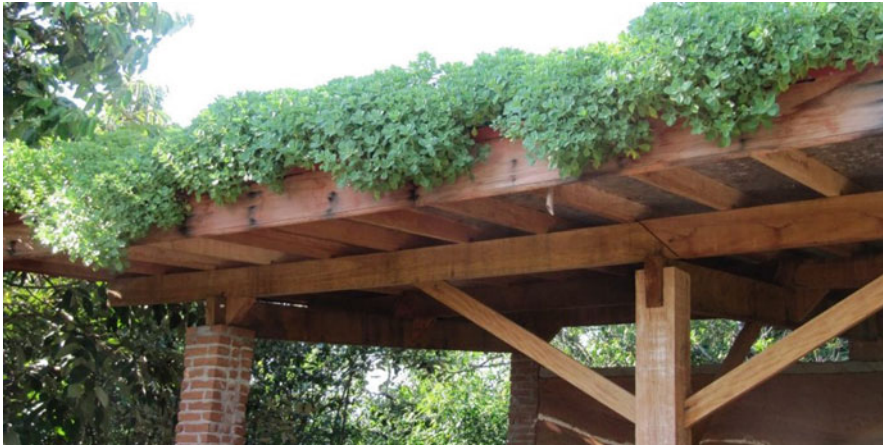
Bio-construction Potential for Sustainability in São Paulo, Brazil, Fig. 7 Green roof. (Source: The authors 2017)
