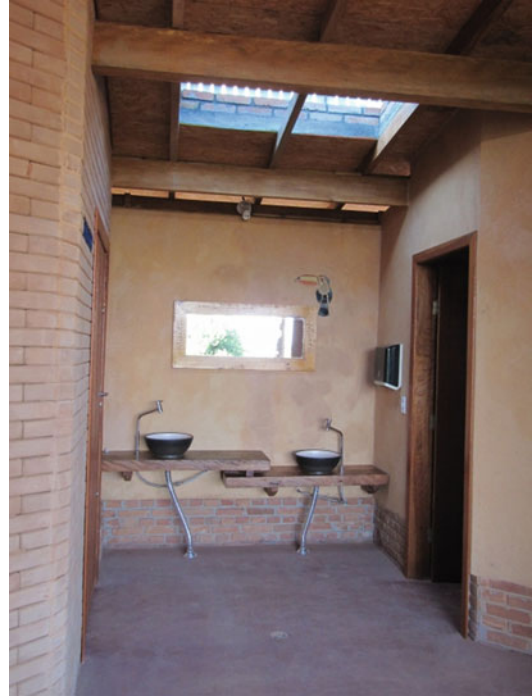
Bio-construction Potential for Sustainability in São Paulo, Brazil, Fig. 4 Zenithal opening. (Source: The authors 2017)
