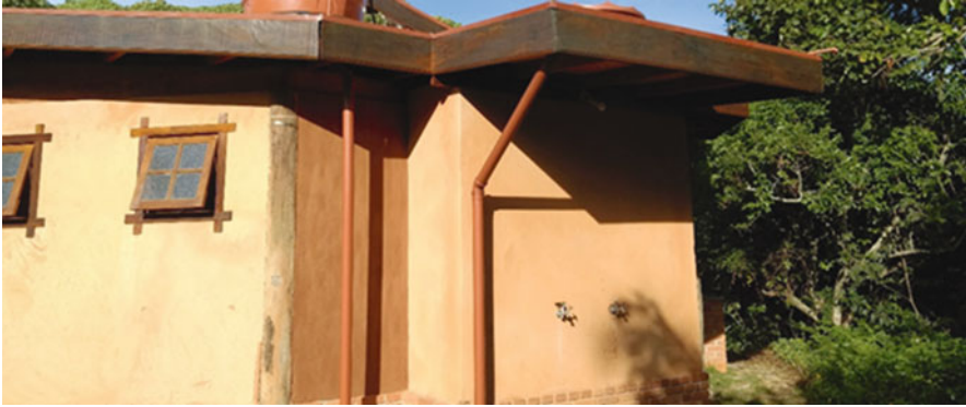
Bio-construction Potential for Sustainability in São Paulo, Brazil, Fig. 5 Rainwater capture. (Source: The authors 2017)
