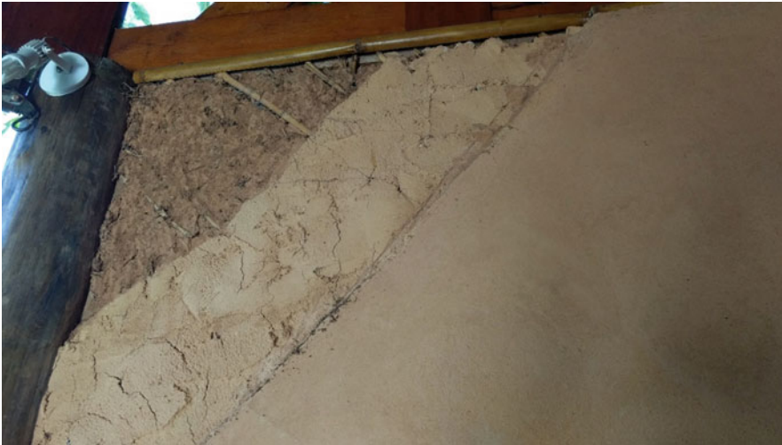
Bio-construction Potential for Sustainability in São Paulo, Brazil, Fig. 2 Mud wall. (Source: The authors 2017)
