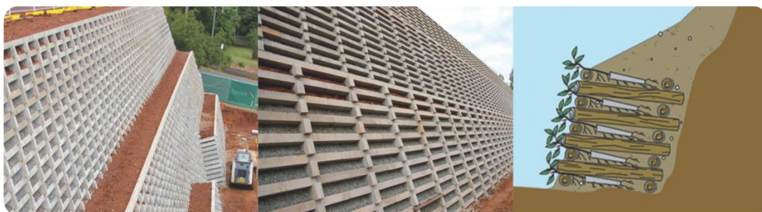
Figura 10– Muro Cribwall
